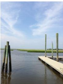
The current condition of the dock and boat ramp at the Marina has been evaluated. While the dock construction is not ideal and the resulting dock not as stable as it might be, it is generally in satisfactory condition for a 30 year old dock and floating pier, with the exception of the ramp lacking handrails. The boat launching pavement pad needs major repairs or replacement because routine use coupled with the brisk Cape Creek tidal current has caused concrete sections of the ramp to separate.
